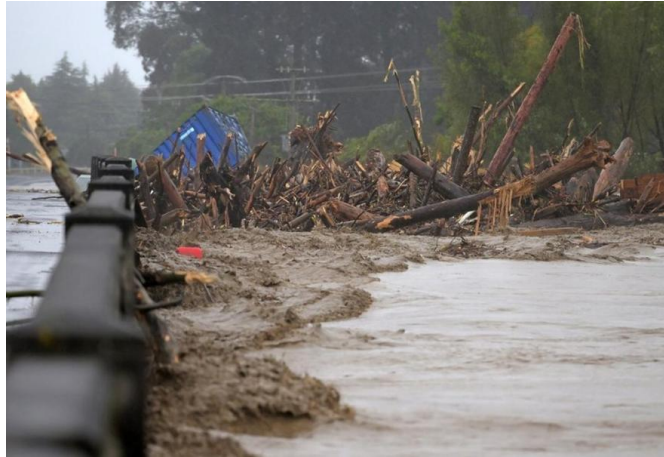
Cyclone Gabrielle flood damage
