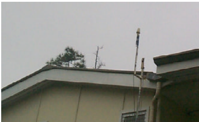
Figure 1: SOPAC GPS base station antenna on top of the MRD building in Mead Rd., Suva. The trees are visible in the background.
