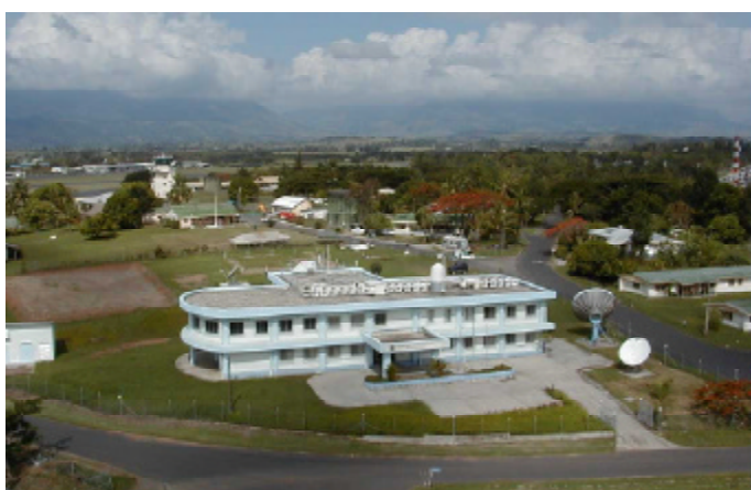
Figure 1: The Fiji Meteorological Building in Namaka, Nadi
