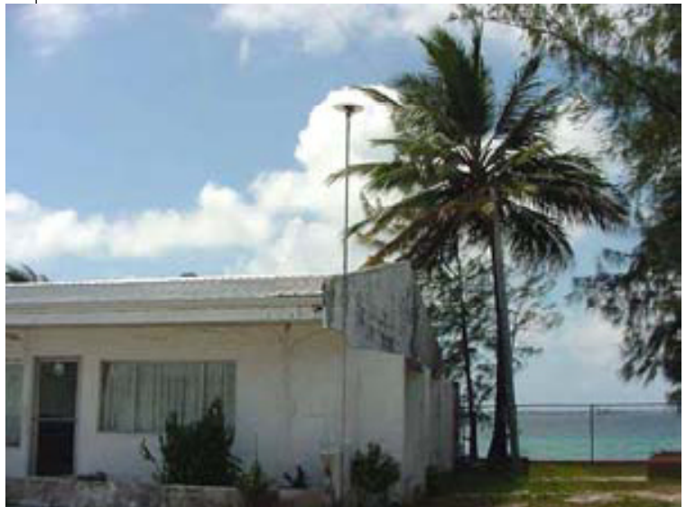
Figure 3: EPA building with GPS antenna
